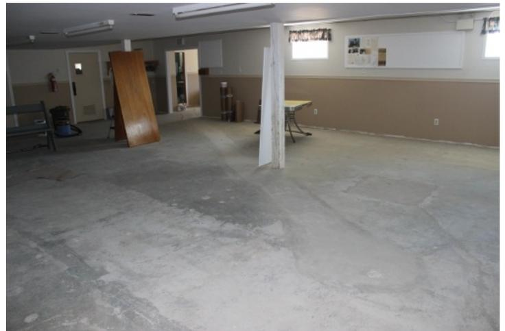
This picture shows the Church Hall where the original concrete floor had to be cut to allow access to the drain beneath, which runs diagonally towards the doorway. Here the new pipe is in place, the trench filled in, and the broken cement floor replaced ready for tiling.
