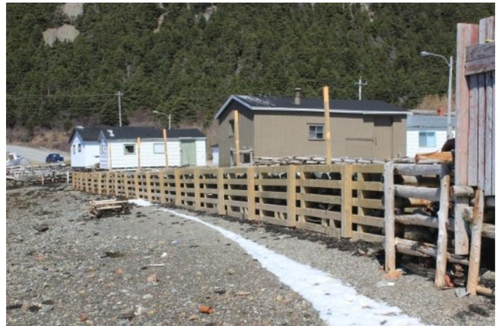
This picture shows the completed breakwater near the junction of Main Street and Park & Youden Road. Solid lumber has been used to build caissons, which were then filled with rock.
